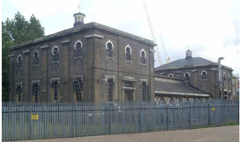
Deptford pumping station Rory Walsh © RGS-IBG Discovering Britain
