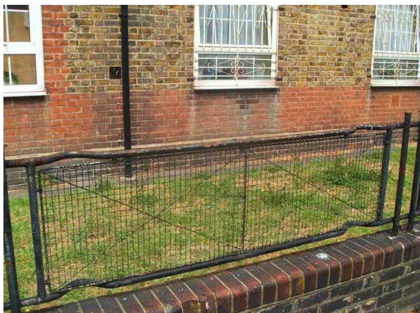
Railings at Rowley House – recycled stretchers Rory Walsh © RGS-IBG Discovering Britain
